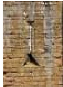
Fishtail arrow loops give space for the crossbow while providing protection for the archer.
